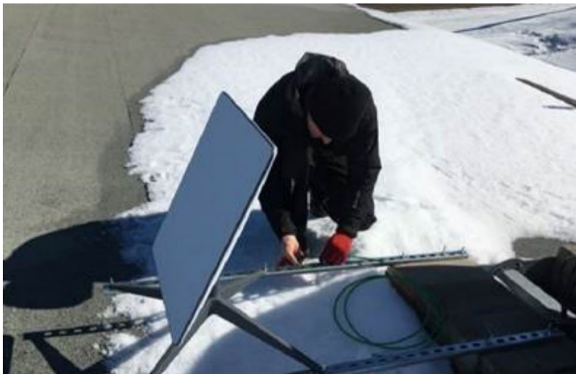
Installation of Starlink satellite system
